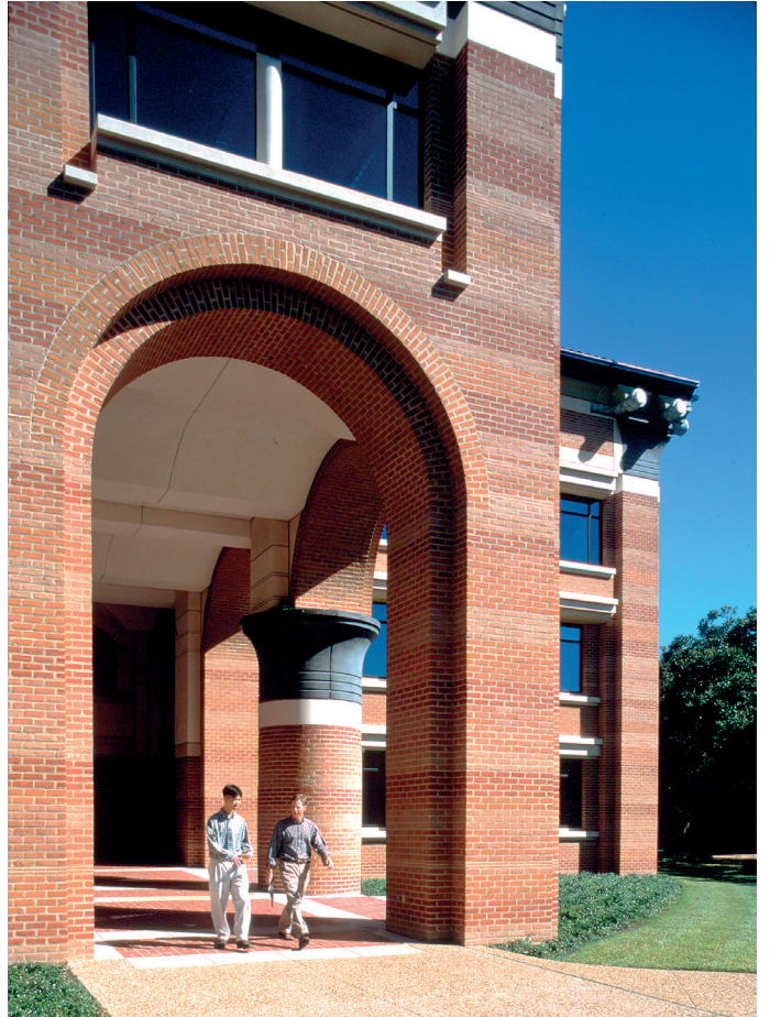
The other extremity of the 300'0" (100M) - long Arcade faces West - towards the main body of the Campus buildings. The Arcade vaulting is plastered so as to look 'internal', and therefore welcoming. It also gives a white surface for the decoration that will come when its conceptual function is appreciated and understood. The curving edge of the 'ground-cover' discs can be seen.
