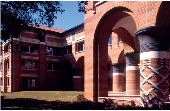
The Arcade alternates round and square columns. This makes diagonal enfilades on a square, hypostylar, grid.
