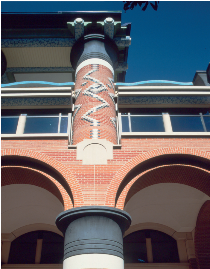
The Tumbling Stream and Confluence fall to the Lazy River over the Balcony of Appearances of Meeting Room 1.
